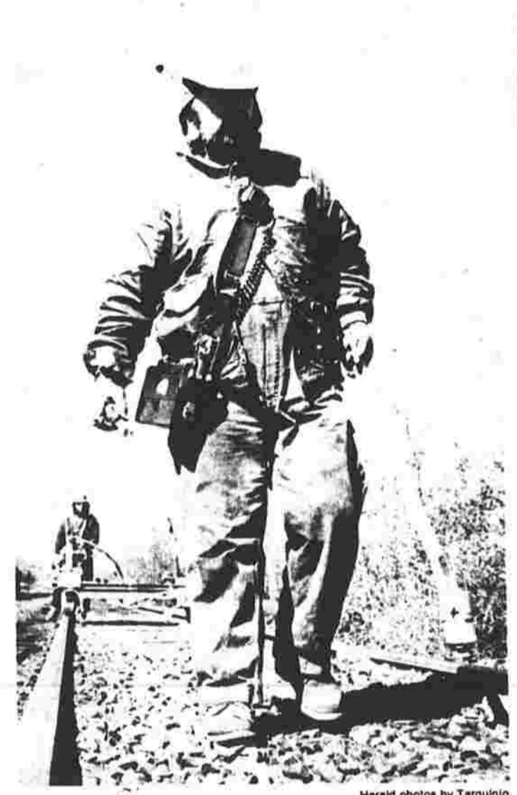
Working on the railroad
